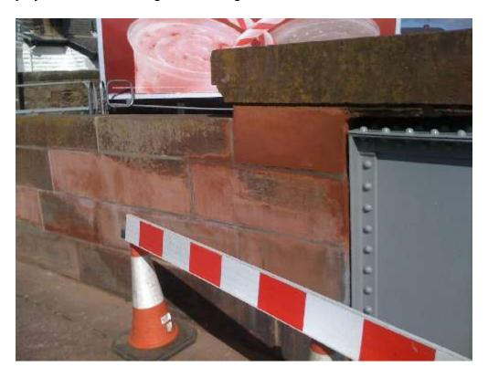
Additional work included repairs to spalled stonework in Lithomex mortar supplied by Mason's Mortars to match the deep red sandstone used in the original construction. Finally the stonework was re-pointed. The work was carried out during the coldest winter and heaviest snow falls seen in Edinurgh for 30 years. Value approx £50,000. Contract supervisor was George King Edinburgh City Council.
