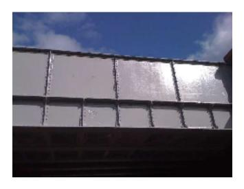
A contract for Edinburgh City Council to blast clean and repaint two Victorian iron bridges carrying roads over a disused railway line in the Lochend district of Edinburgh. Blast cleaning carried out to Sa21/2. The coating system was RT98 epoxy primer, underocat and polyurethane finish. The parapets were finished with PPG's PSX700 polysiloxane as an anti-graffiti coating.
